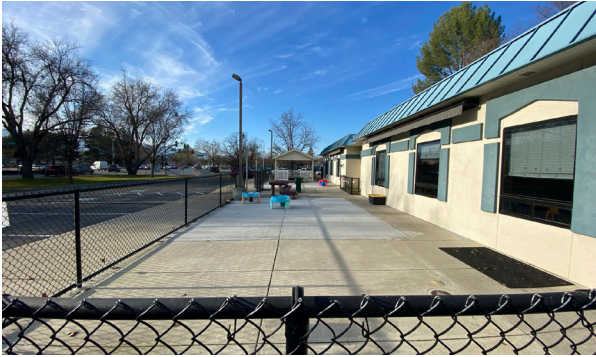
Front Entry and Outdoor Classroom
