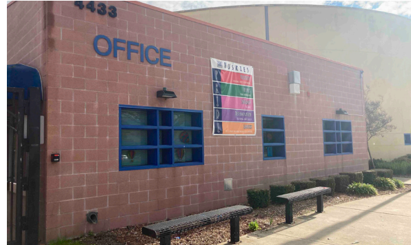
Front Office / Main Entry
